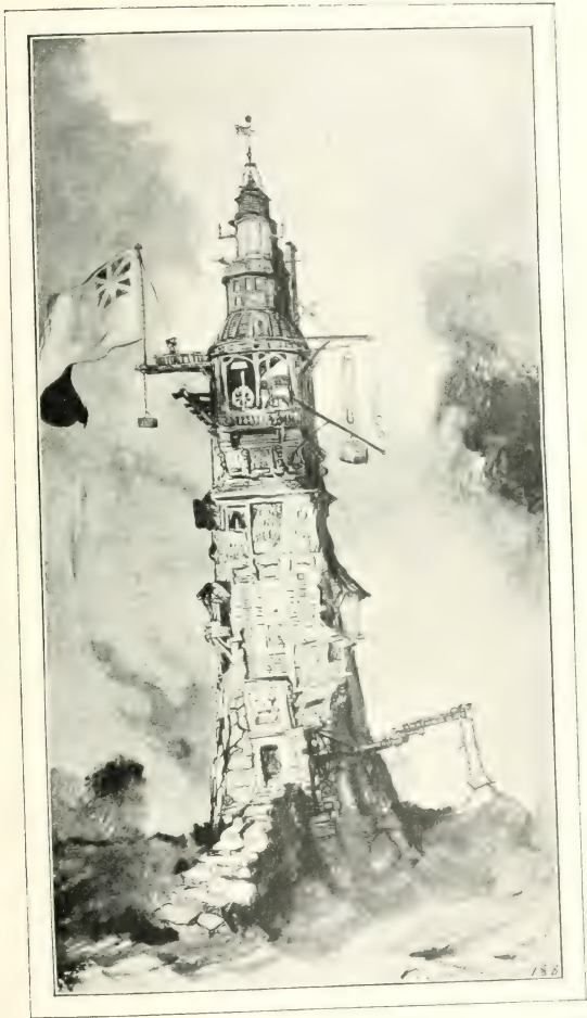
THE LIGHTHOUSE CONSTRUCTION
